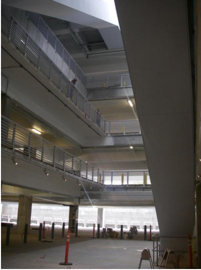
RCF CSB Escalator Openings Paint/Lighting
